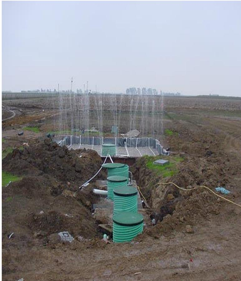
*Photo shows the squirt test for an alternative OWTS using a sand filter system as a pretreatment prior to the disposal field*
