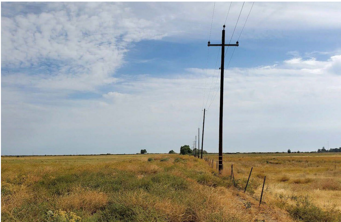
Photo 8. Existing utility line in northern portion of Project Site (to be removed) (August 5, 2022)
