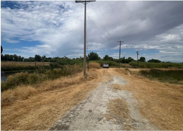
Pole #9 and pull site
