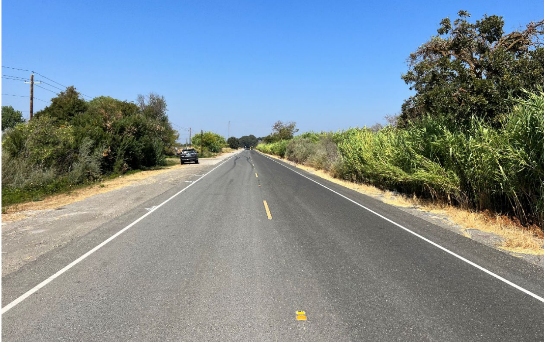
Photo 9. Existing utility line in northern portion of Bank property (August 31, 2023)
