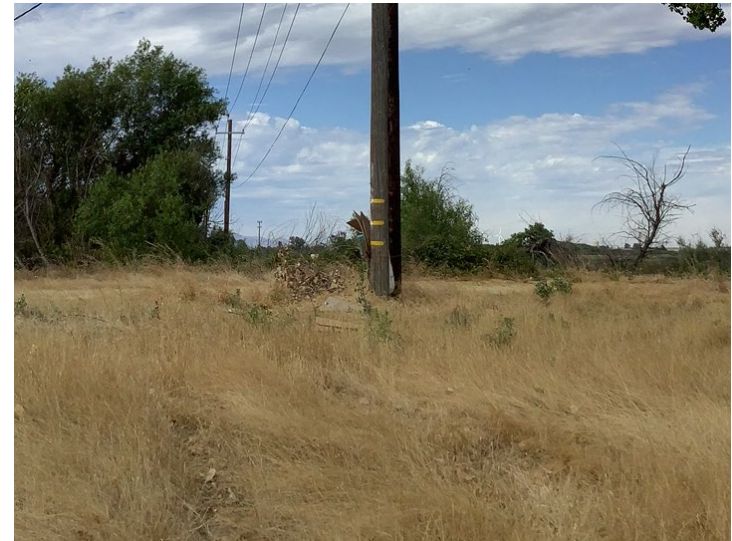
Pole #10 (near Highway 84)
