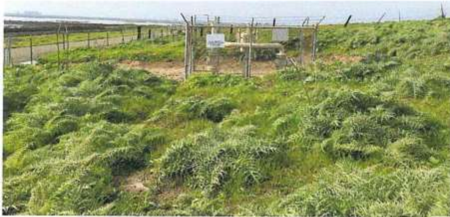
Proposed pipeline tie-in point. View looking west from east side of pipeline tie-in point.
