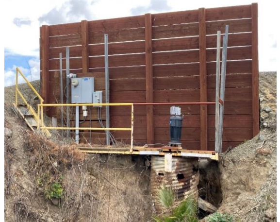
Collinsville Levee Pump – After Repair Winter 2022
