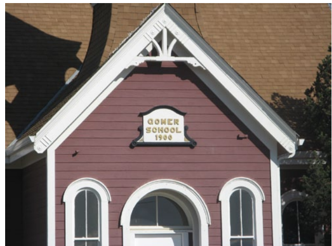
Gomer School reflects the architectural detail of the early 20th century.
