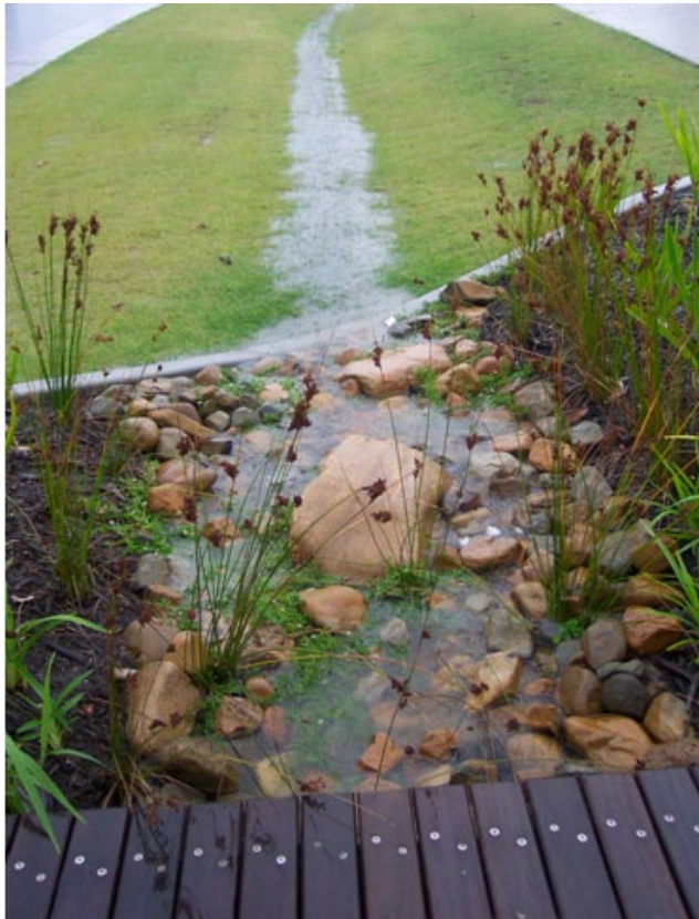
Open channels in the street right-of-way should be used to convey and treat stormwater runoff.
