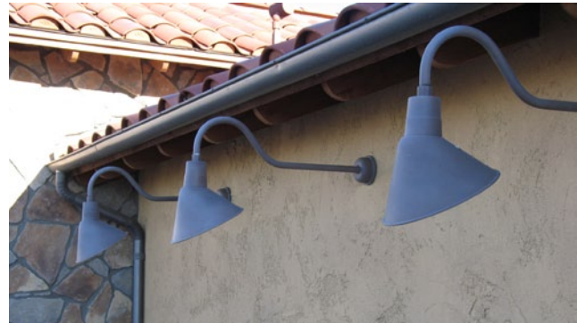
Light fixtures should be located at regular intervals to maintain a smooth, level lighting intensity.
