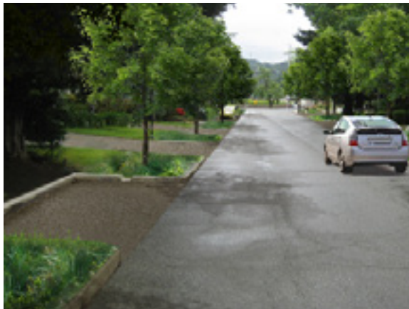
Parking areas utilize pervious solutions as feasible
