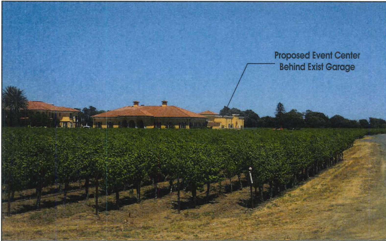
EXISTING 8,000 SQ. FT. PRIVATE GARAGE, MAIN HOUSE TO THE LEFT, PROPOSED EVENT CENTER IS BEHIND.
