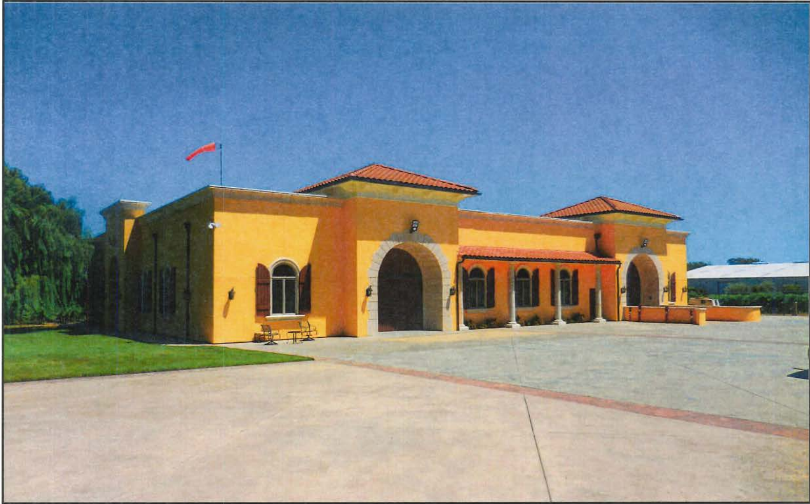
EXISTING 12,000 SQ. FT. STORAGE BUILDING
