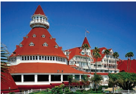
Hotel Del Coronado Historic Renovation, San Diego
