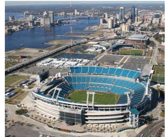
Alltel Stadium Jacksonville, FL Renovation of Gator Bowl
