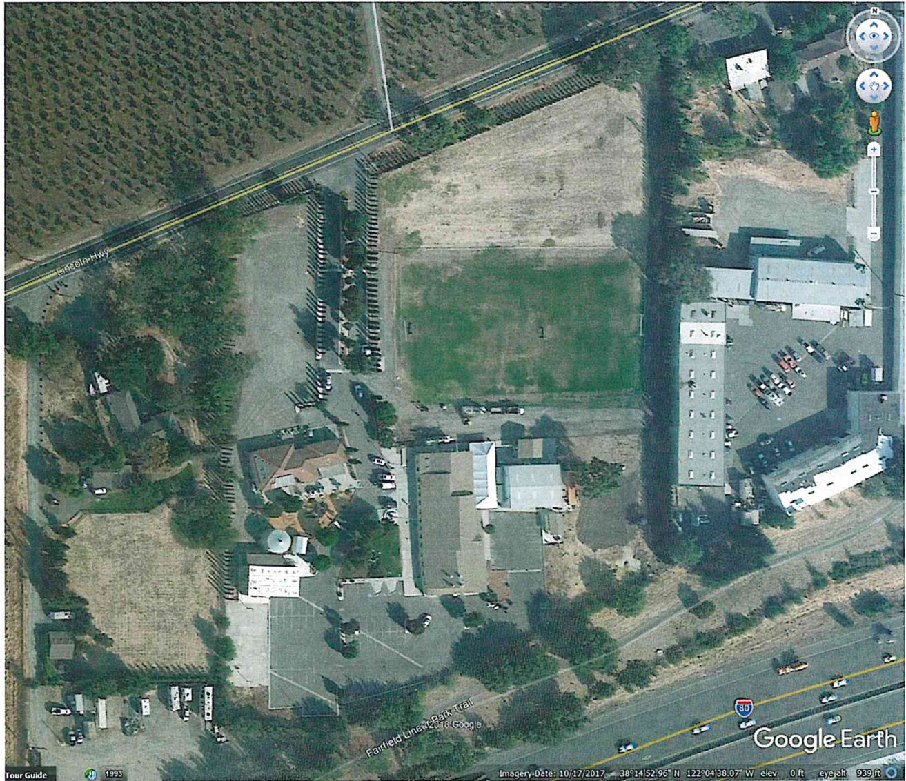
Figure 3: Aerial Photo Project Site – October 2017
