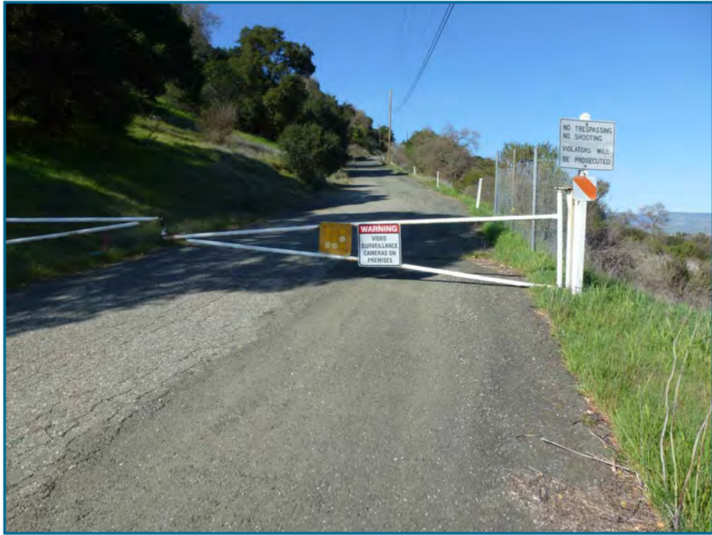
Photograph 1 - Locked entry gate.
