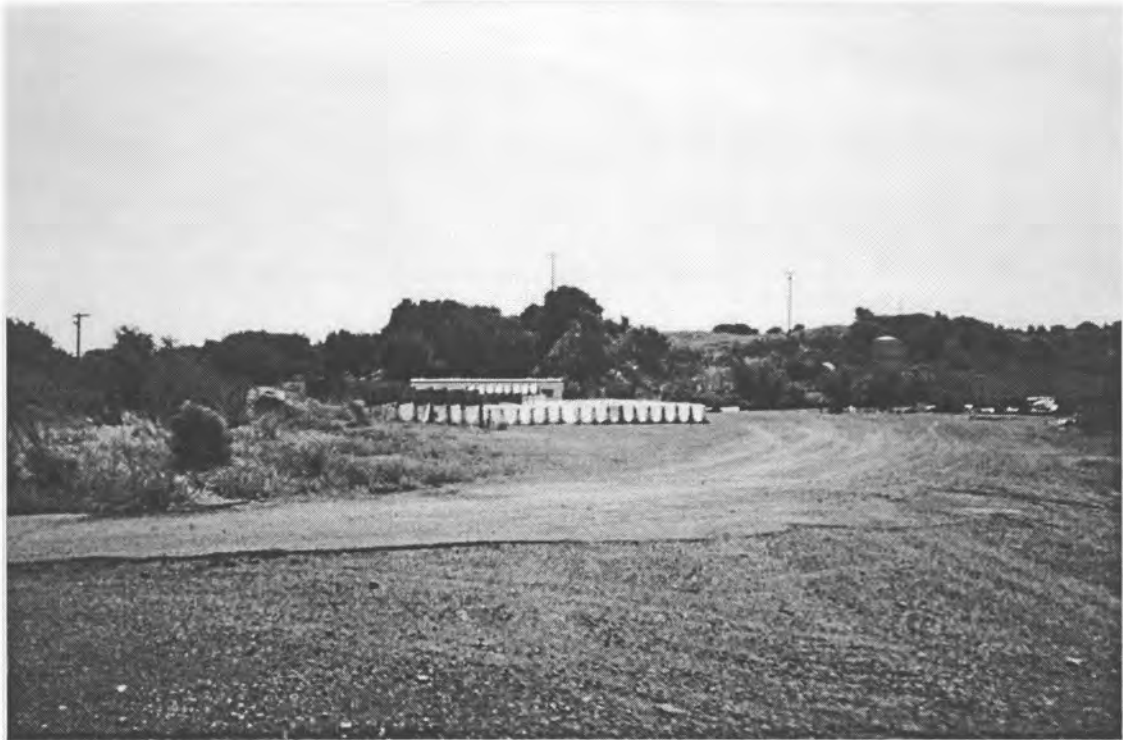
Access and Staging Area
