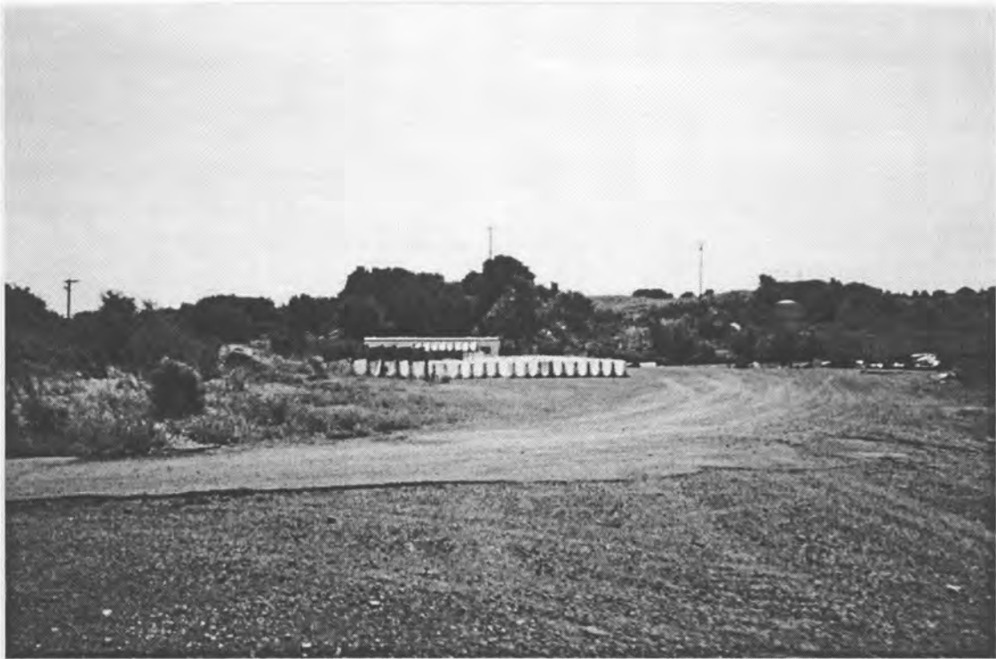
Access and Staging Area
