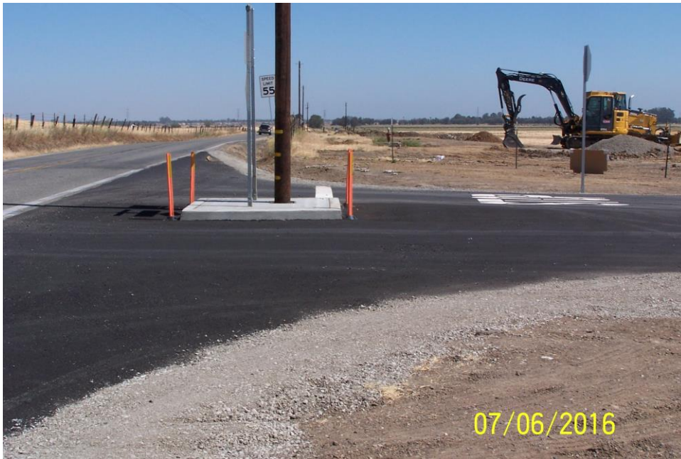
Photo 3 - View looking north at new access connection to North Gate Rd.
