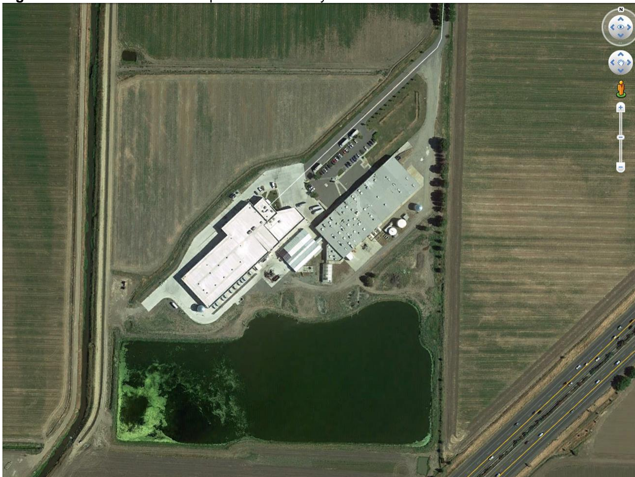
Figure 2: Aerial Photo of Site Improvements – May 2017
