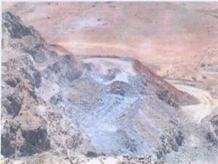
Detail of benches and recently blasted material.
