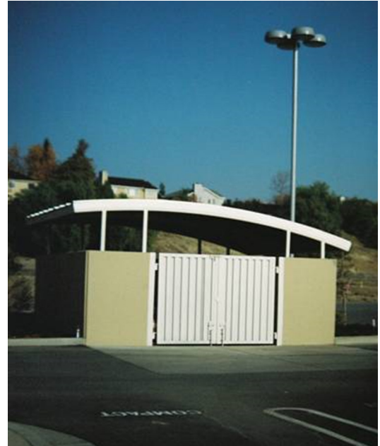
Figure 3.1. Roofed and bermed refuse area.
