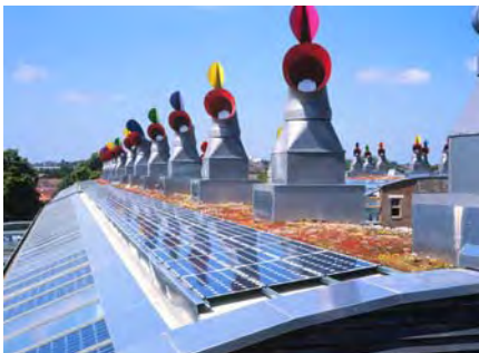
Beddington Zero Energy Development, UK
