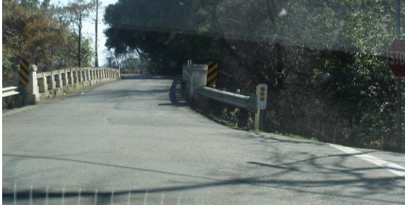
Existing Bridge on Suisun Valley Road
