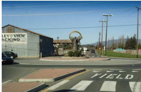
Existing roundabout at Abernathy and Rockville Roads
