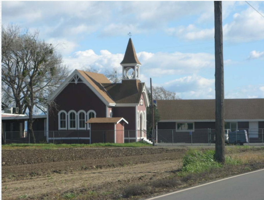
Front and side gabled roofs are typical.
