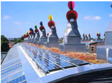
Beddington Zero Energy Development, UK
