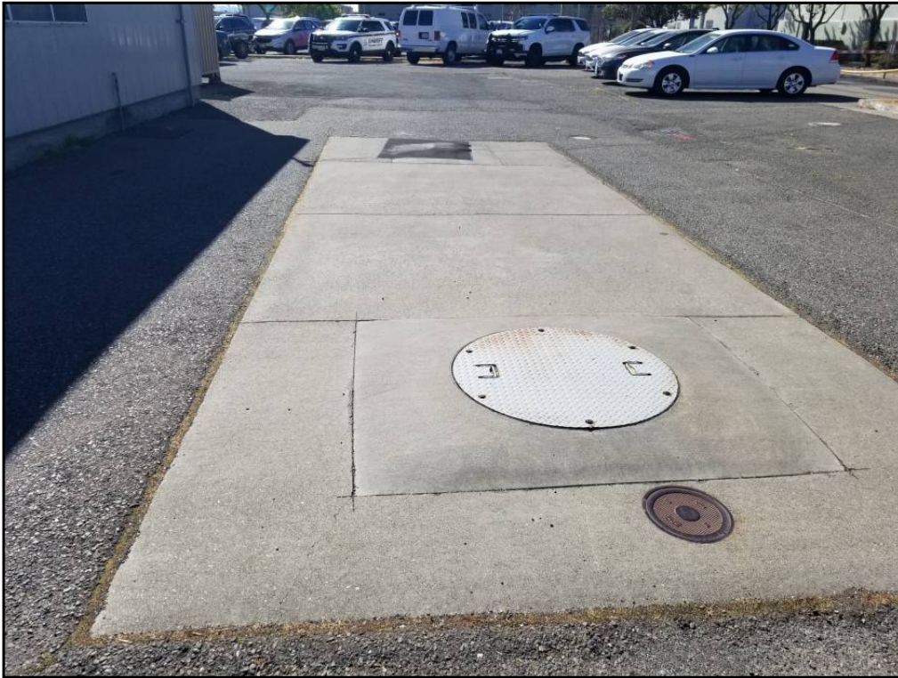
37 : View of the 10,000-gallon gasoline UST.
