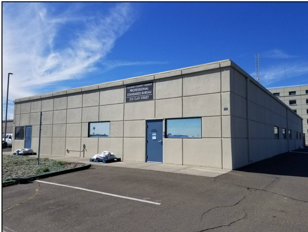
50 : View of the exterior of the General Services building (510/512 Clay Street).
