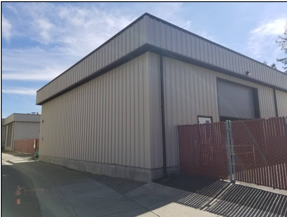
60 : View of the exterior of the storage building (509 Delaware Street).
