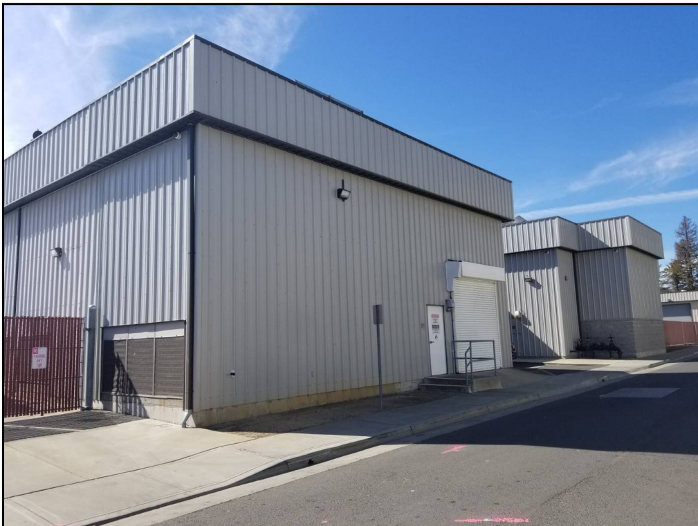
52 : View of the exterior of the Co-Gen Plant (501 Delaware Street).
