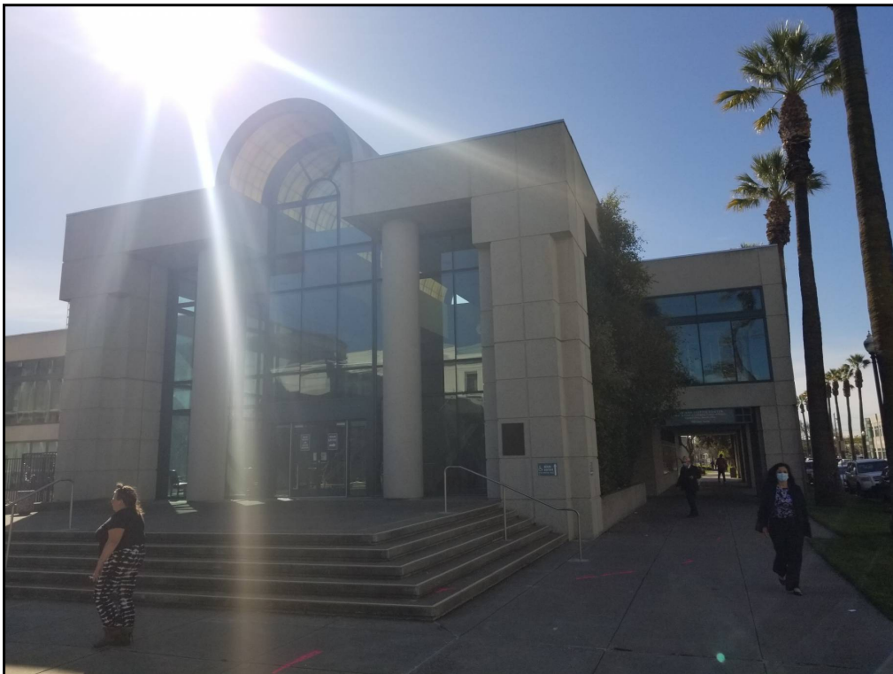
6 : View of the exterior of the Law and Justice Center (530 Union Avenue).
