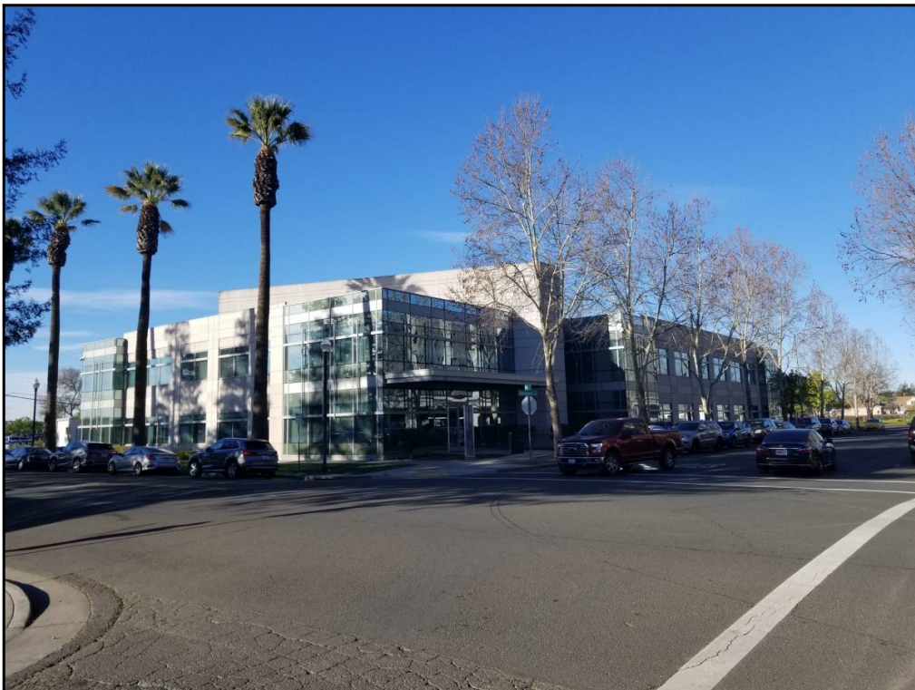
90 : View of the Solano County Probation Department (475 Union Avenue) to the west of the site.
