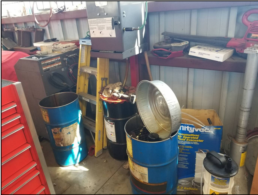
41 : View of the oil filter crushing station. No signs of leaks or spills were observed.
