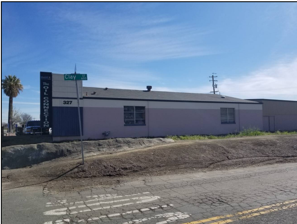
80 : View of 327 Texas Street to the east of the site.
