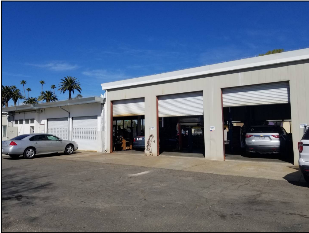
35 : View of the exterior of the Fleet Services building (447 Texas Street).
