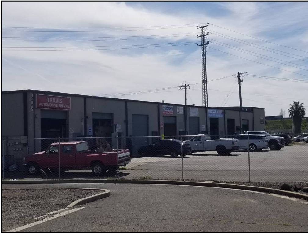
85 : View of 408 Union Avenue to the south of the site.
