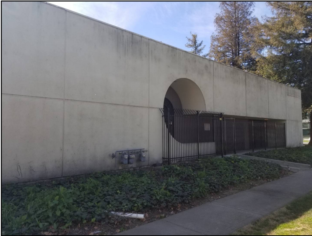
87 : View of 460 Union Avenue, to the west of the site.
