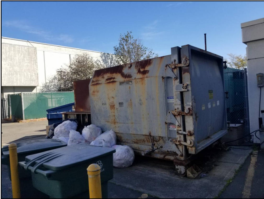
5 : View of the Hall of Justice waste collection area.
