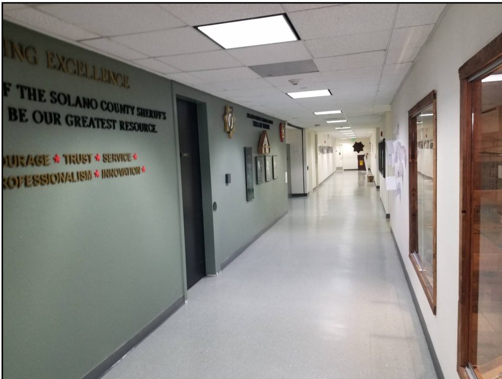
16 : View of a hallway in a site building.
