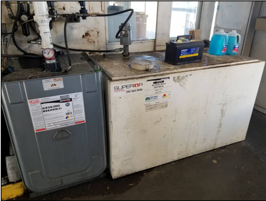
39 : View of the 250-gallon and 110-gallon oil ASTs. De minimis oil stains were observed at the base of the ASTs.
