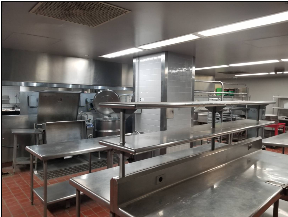
20 : View of the County Jail kitchen.
