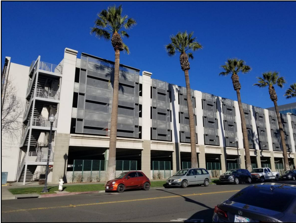
89 : View of the parking garage (531 Union Avenue) to the west of the site.
