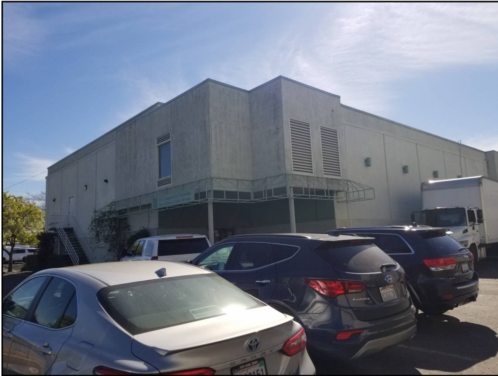
31 : View of the exterior of the UC Co-Op Extension Agricultural building.
