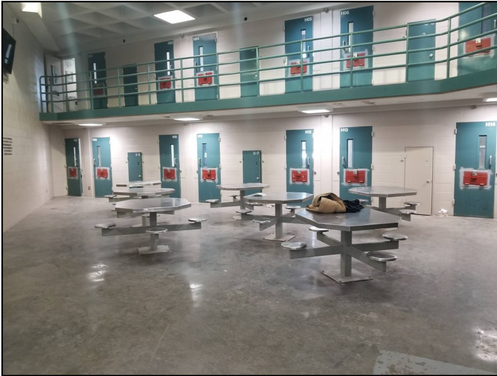
21 : View of a typical modular in the County Jail.
