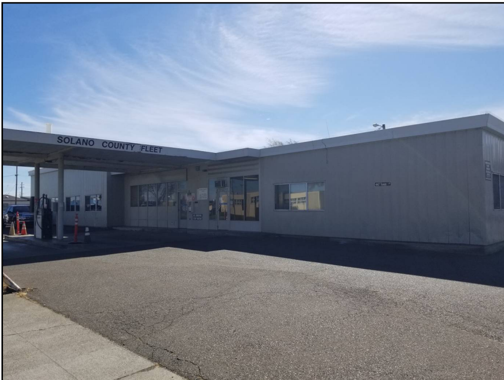
34 : View of the exterior of the Fleet Services building (447 Texas Street).
