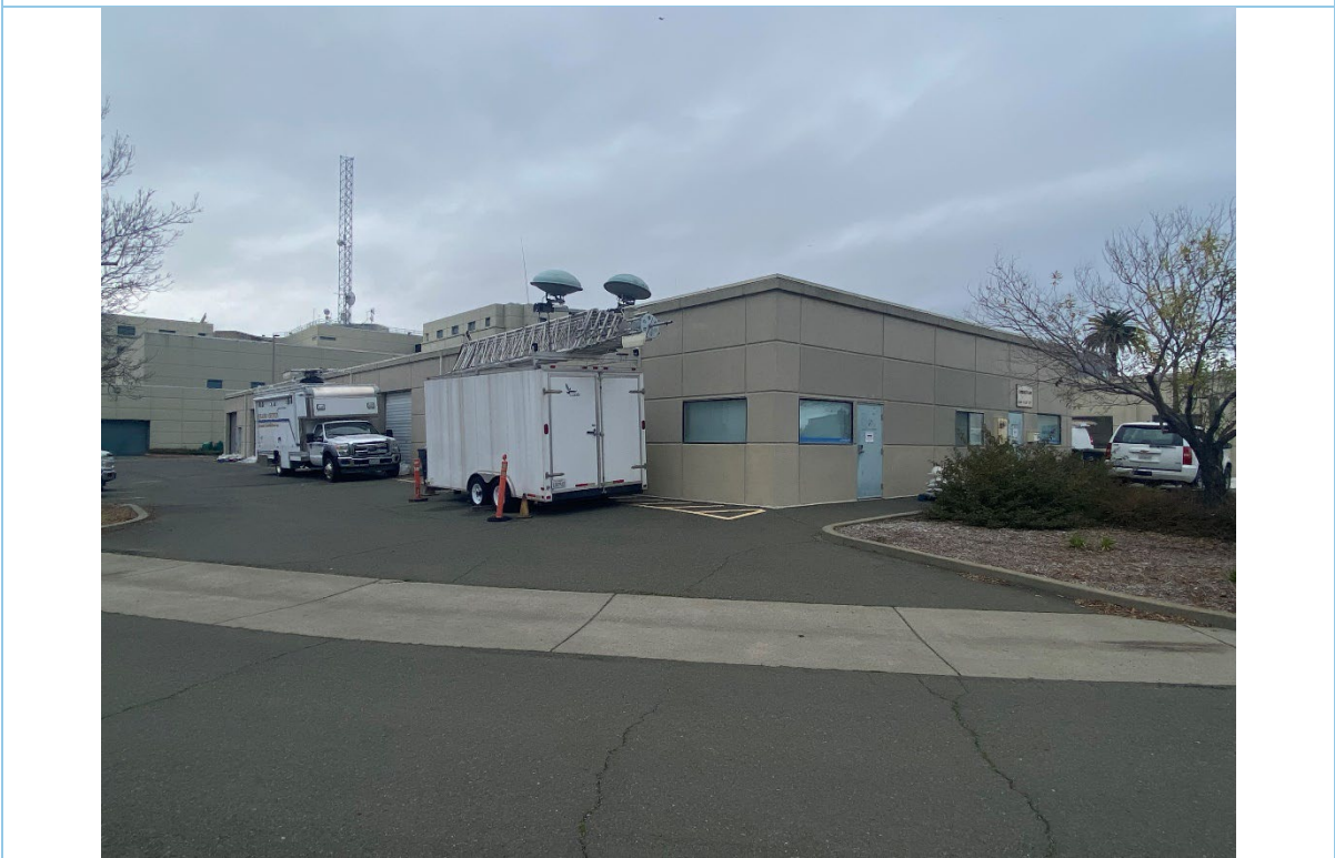
Photograph 2: View from the southeast corner of the project site; facing northwest.
