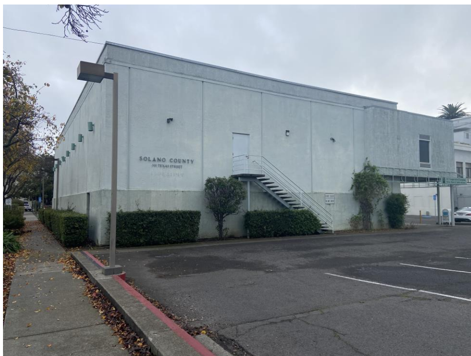
Photograph 5. UCCE/Agricultural Building, north elevation, view southwest.
