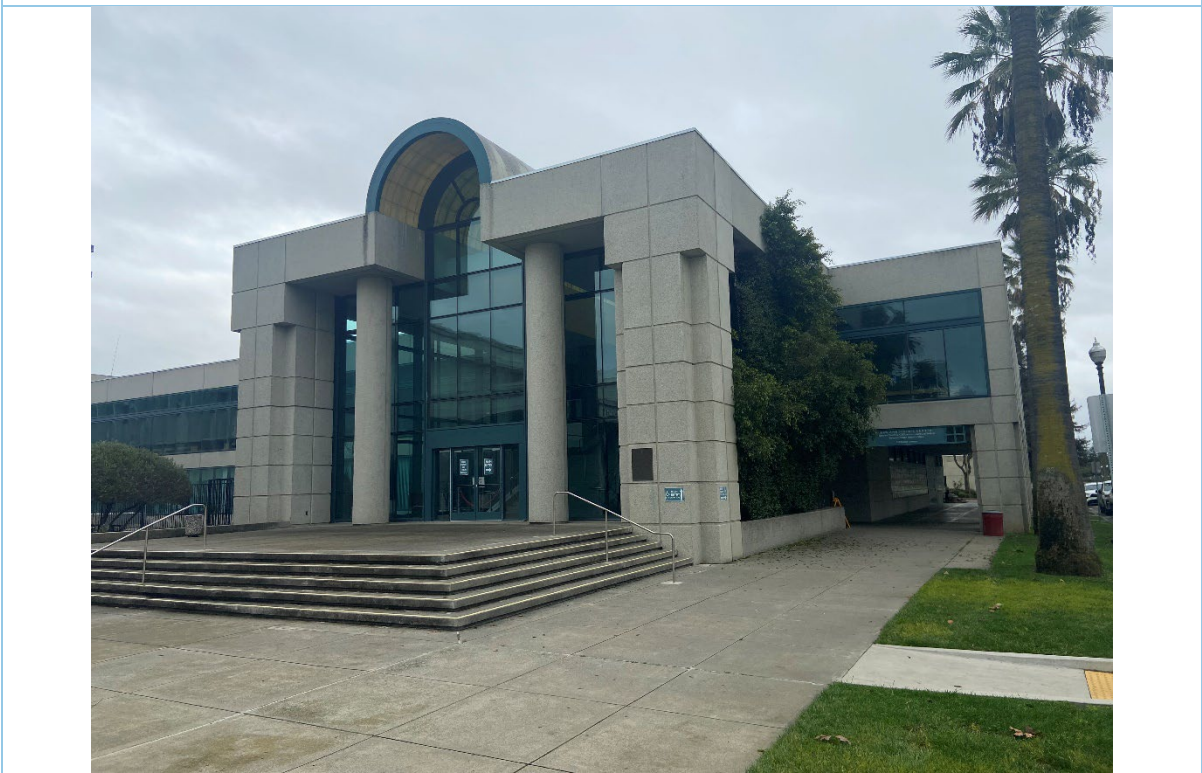
Photograph 6: Detail of administrative office building; facing southeast.
