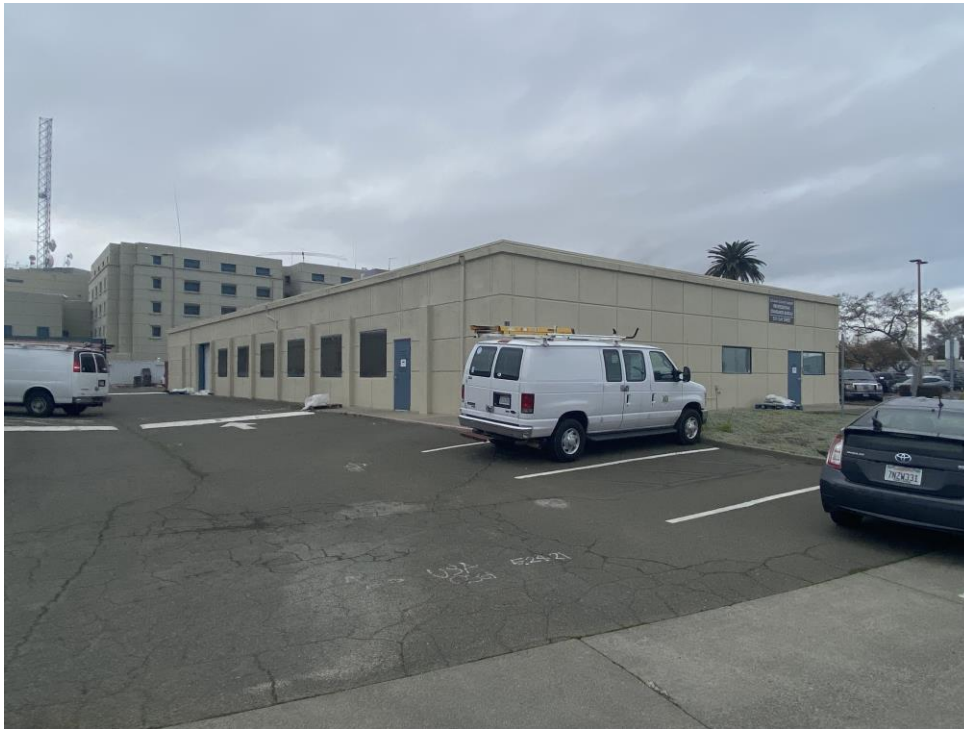
Photograph 2: 510-512 Clay Street, south and east elevation, view northwest
