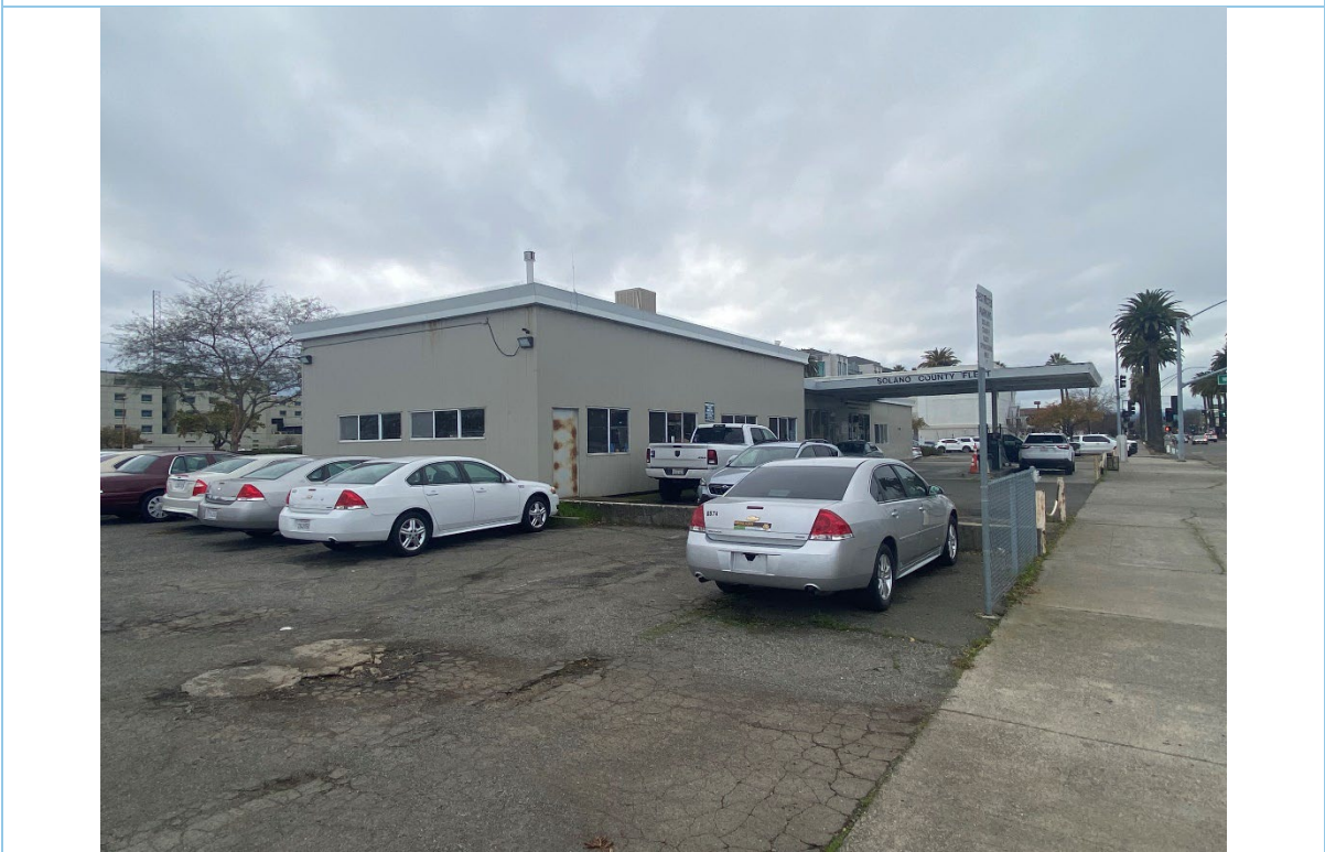
Photograph 10: Detail of Solano County Fleet Services building; facing southwest.
