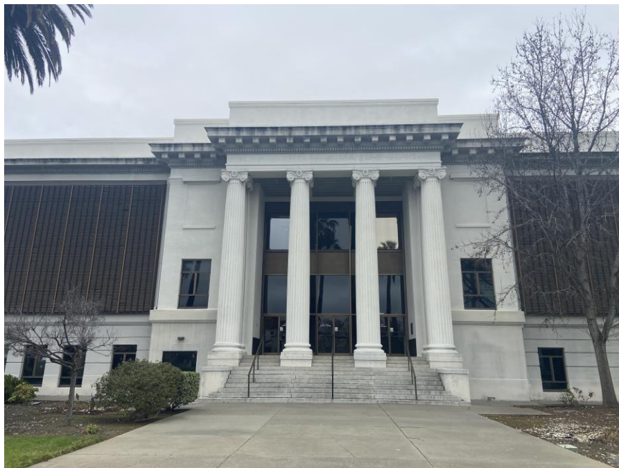
Photograph 3. Primary elevation, front entrance; facing east.
