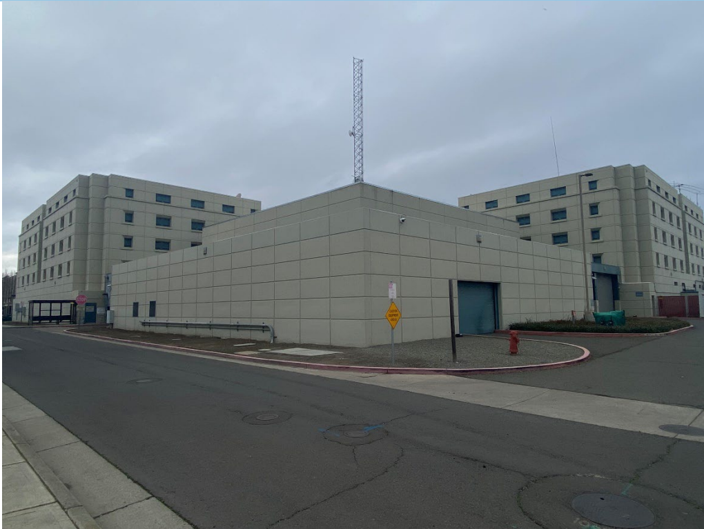
Photograph 7: Detail of county jail facilities; facing northwest.
