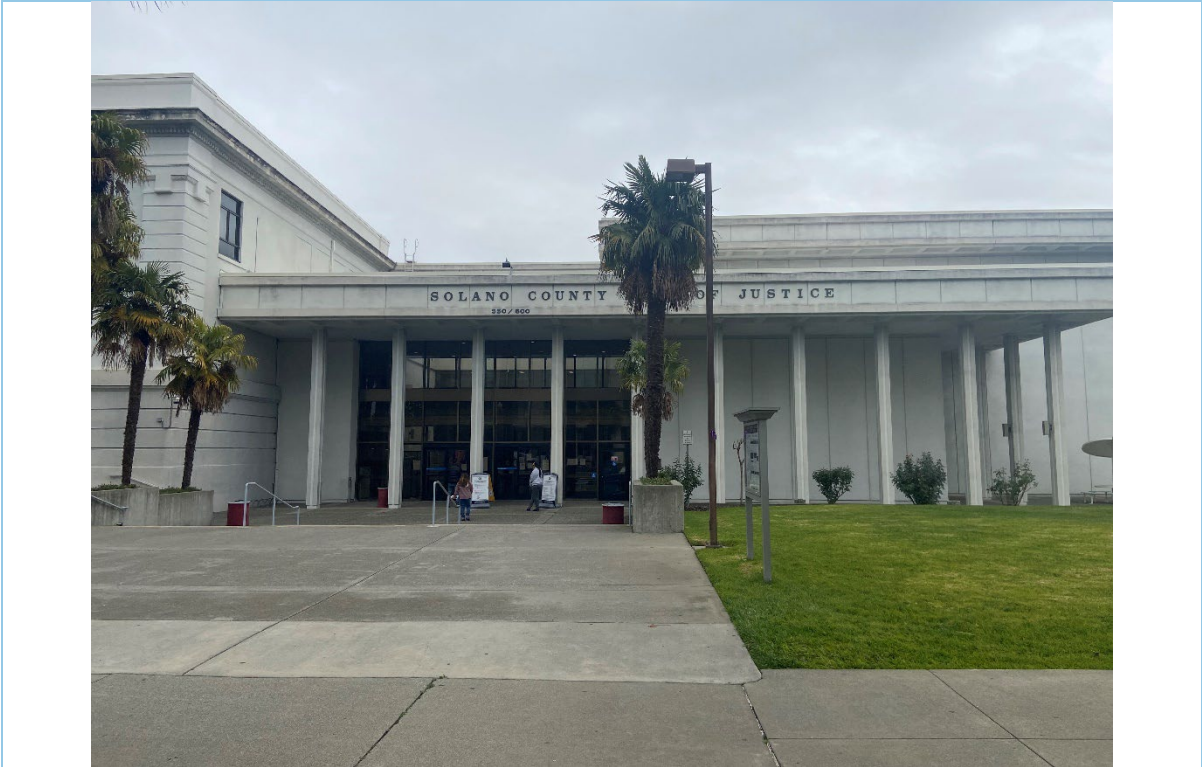
Photograph 5: Detail view of Solano County Hall of Justice II; facing east.
