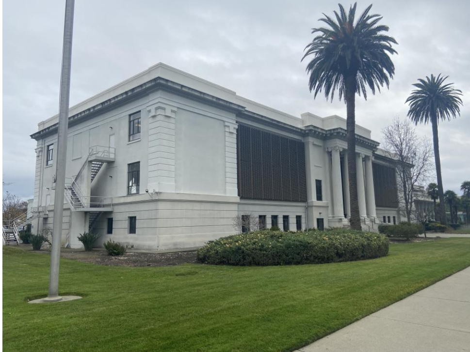
Photograph 2. North and west elevations; facing southeast.
