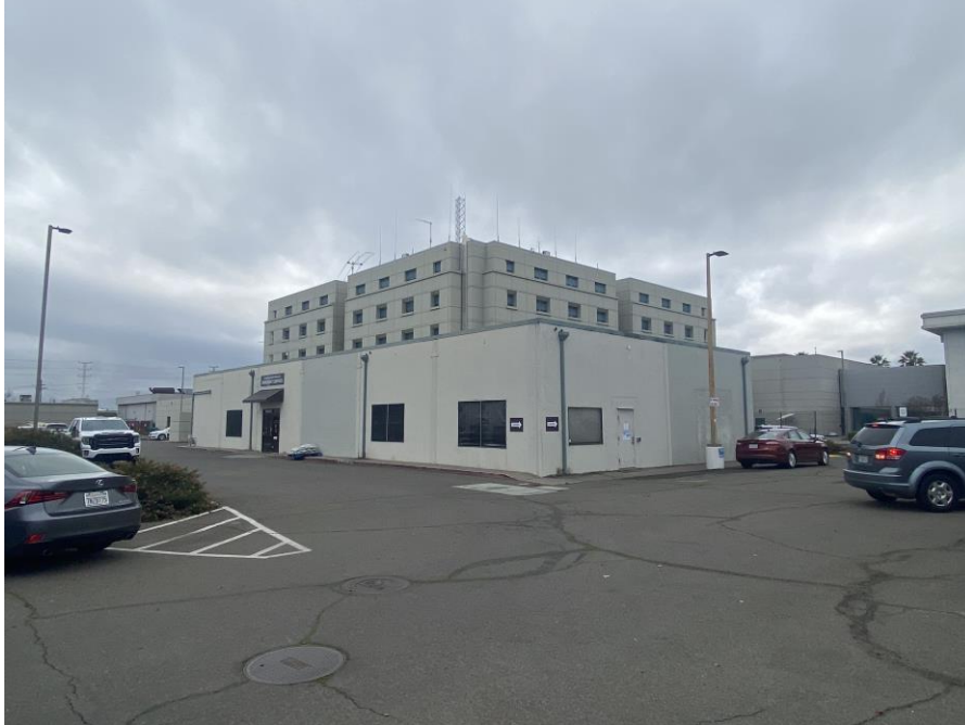
Photograph 3: 530 Clay Street, north and east elevation, view southwest
