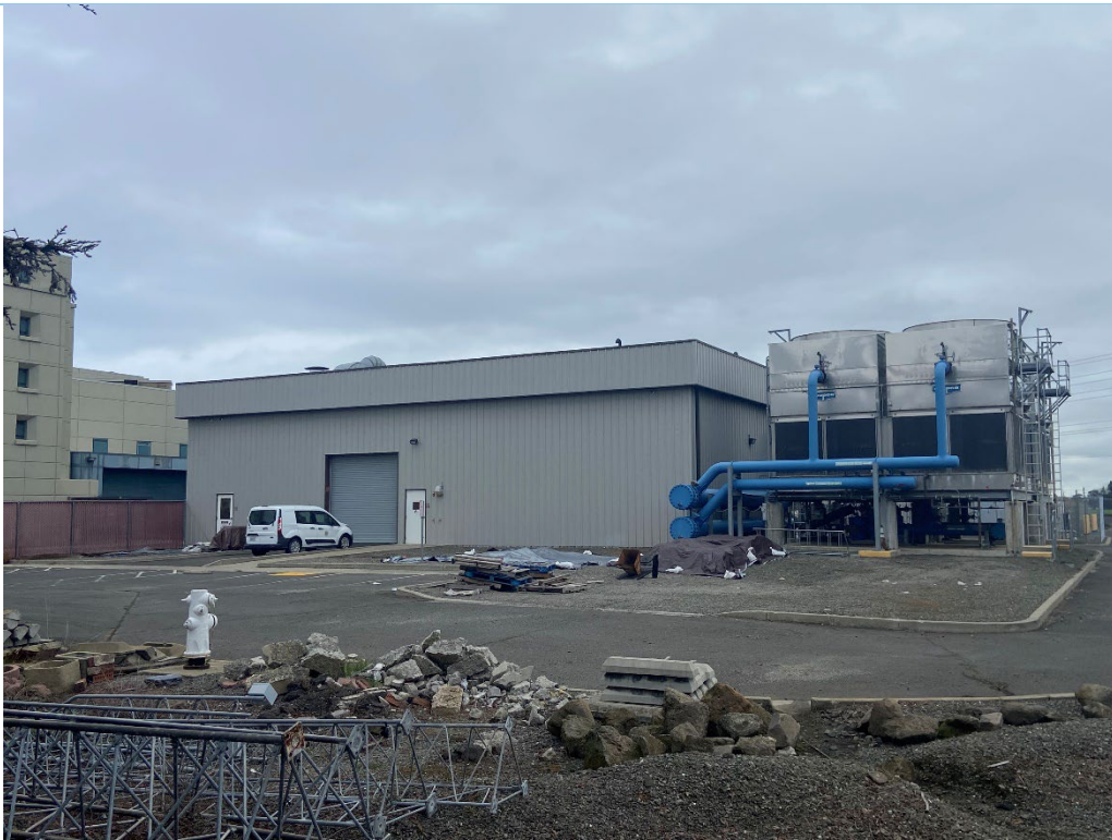
Photograph 8: Detail of physical plant buildings; facing east.
