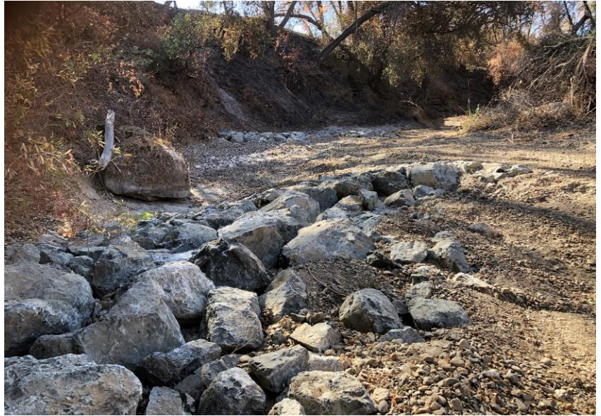
Figure 8-2: Rock Vanes Installed after LNU Fire by SCWA
