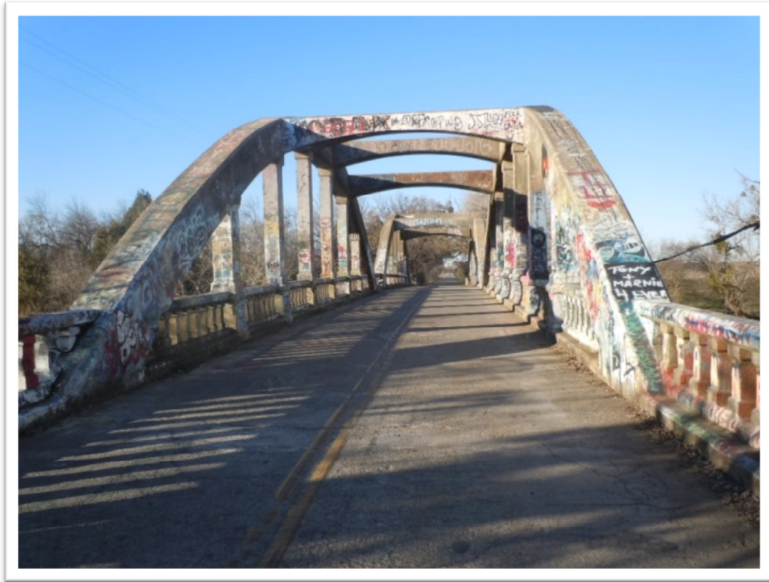
Photo of Stevenson Bridge, looking north
