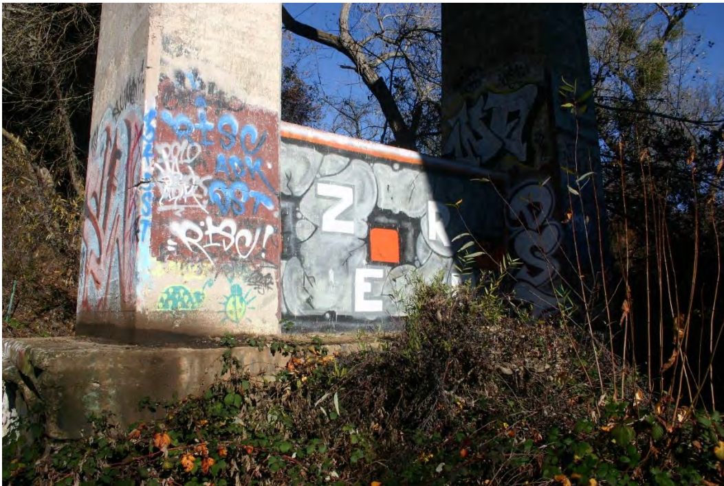
Photograph 8. Footings at pier columns will be retrofitted. Detail view.
