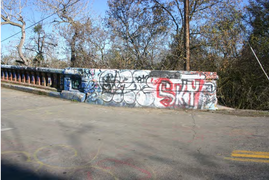
Photograph 5. Solid end posts with incised panels, view facing northeast.
