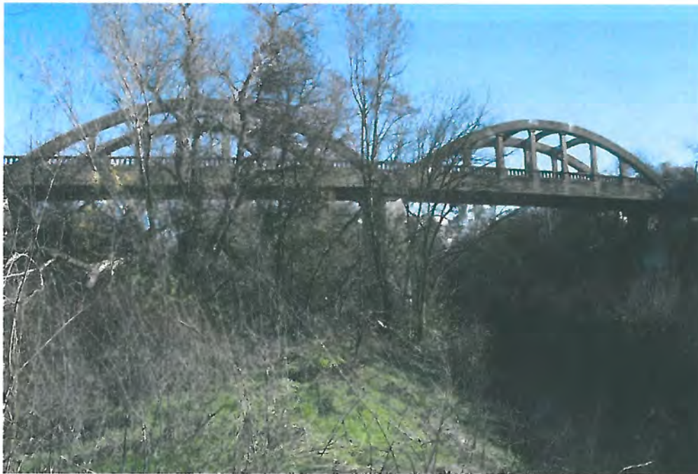
Image 3. West elevation, two-span, reinforced concrete, open spandrel arches, view facing east.
