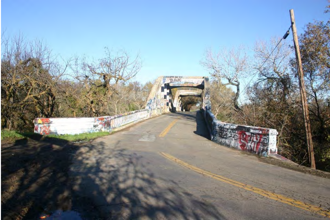
Photograph 1. Overview of south approach to bridge, view facing north.
