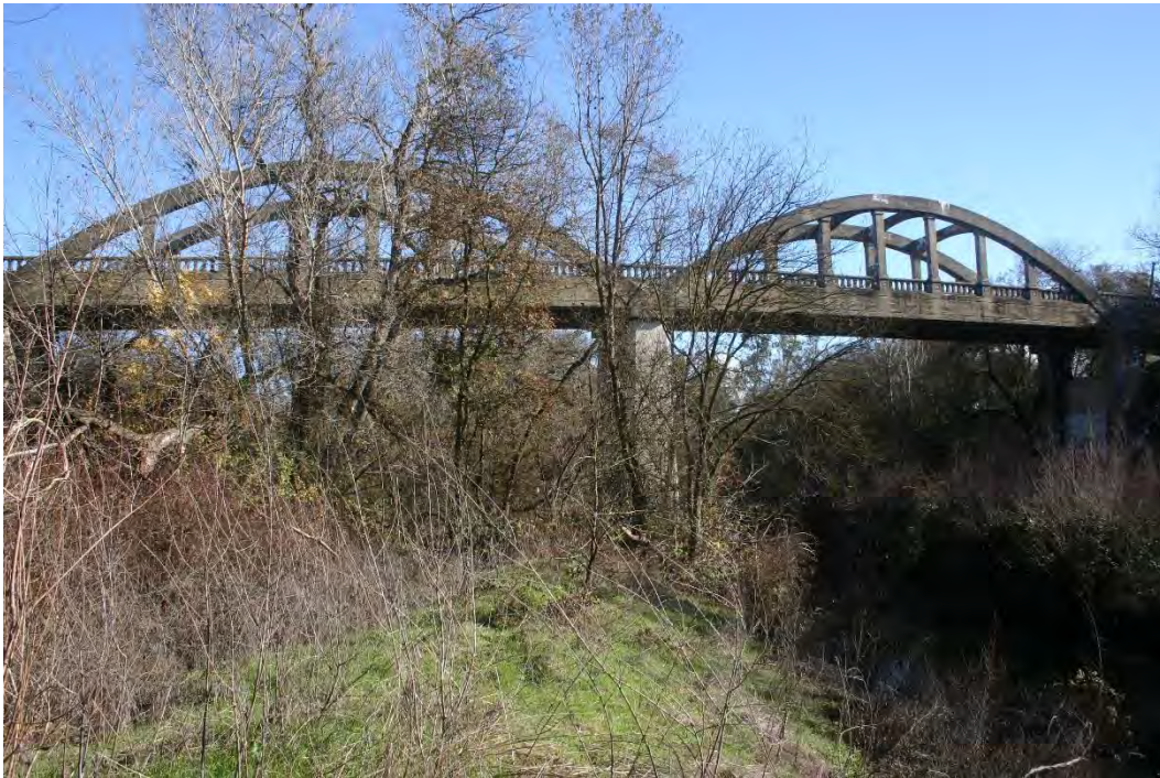
Photograph 2. Elevation of Bridge 23C0092, view facing east.
