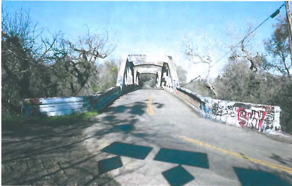
Image 2. South portal and wing walls, view facing north.
