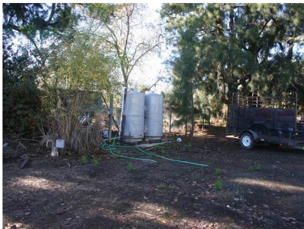
Image 8. Water tanks, view facing southwest
