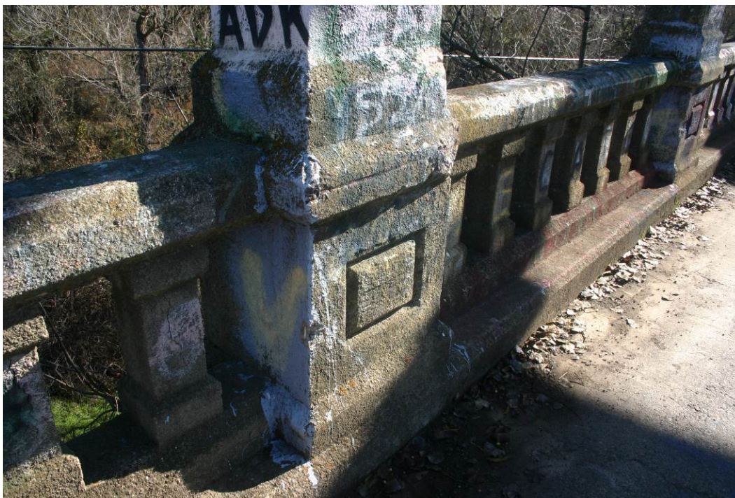
Image 4. Reinforced concrete railing with rectangular window rail design and smooth concrete finish, view facing southeast.
