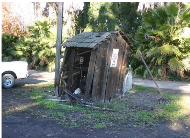
Image 7. Wood frame pump house, view facing northwest
