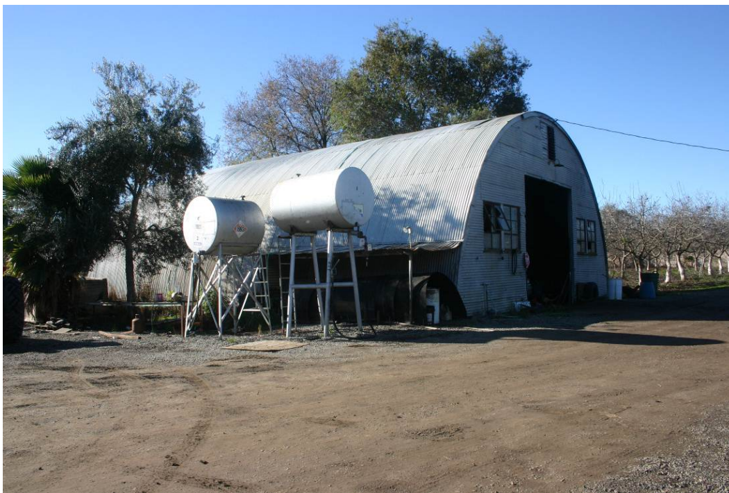
Image 5. Quonset building (c.1945) labeled F on sketch map,, view facing southwest
