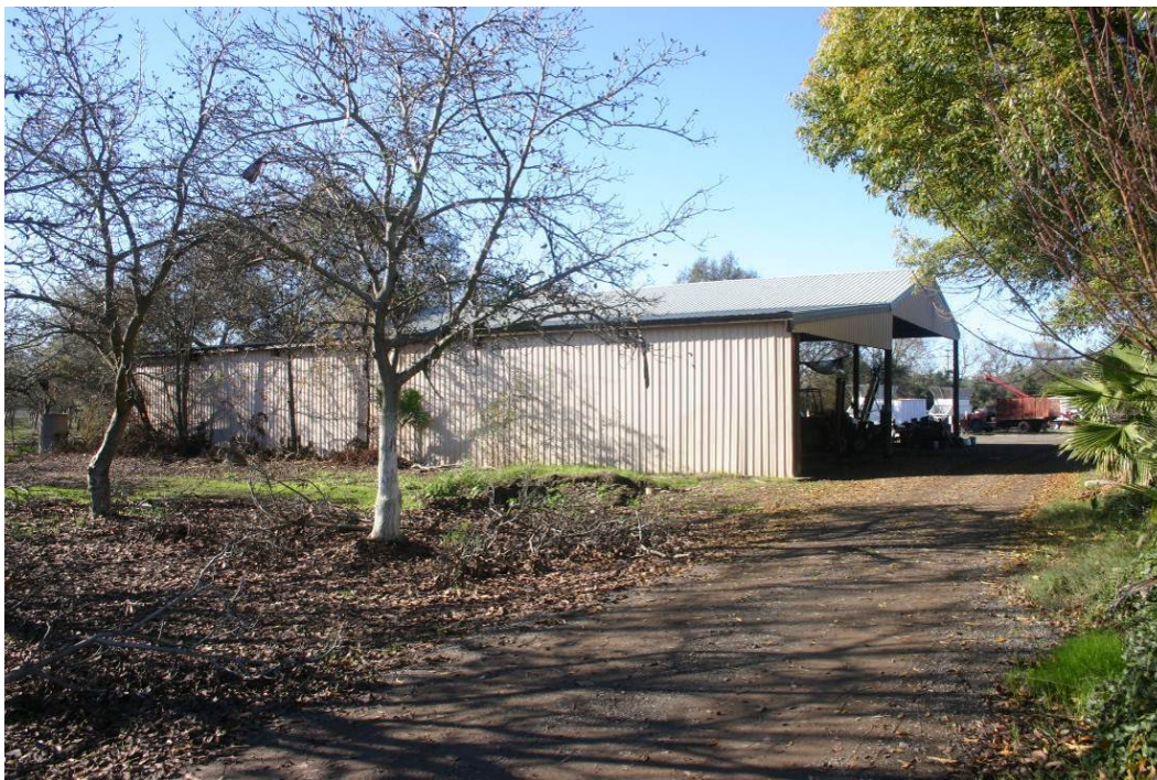
Image 4. Metal pole barn (c.1975) labeled E on sketch map,, view facing southwest
