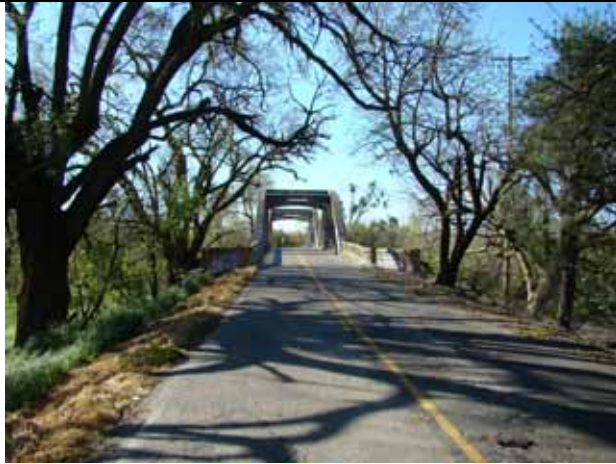
Photo 1: North road approach to Stevenson Bridge. 31 Mar 2011.
