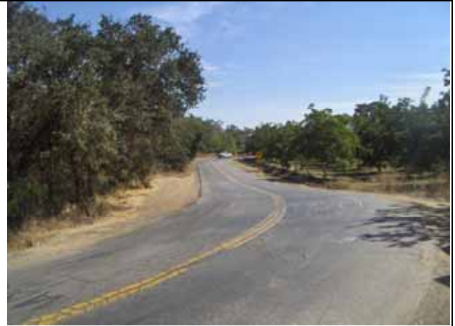
Photo 2: South road approach to Stevenson Bridge. 28 Sept 2009.
