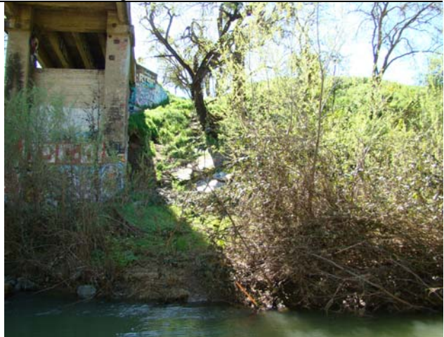
Photo 4: Looking south under Stevenson Bridge. Steep slopes surrounding Putah Creek. 31 Mar 2011.
