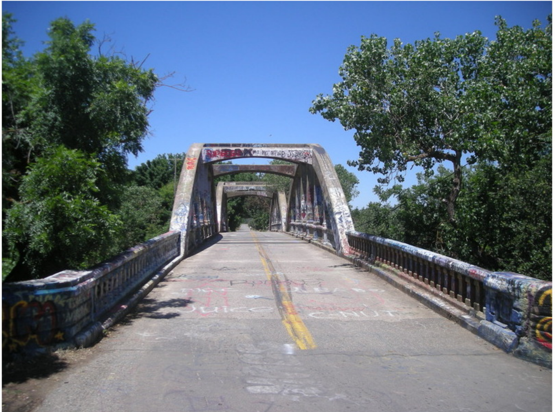
Photo No. 1 Roadway view looking North
