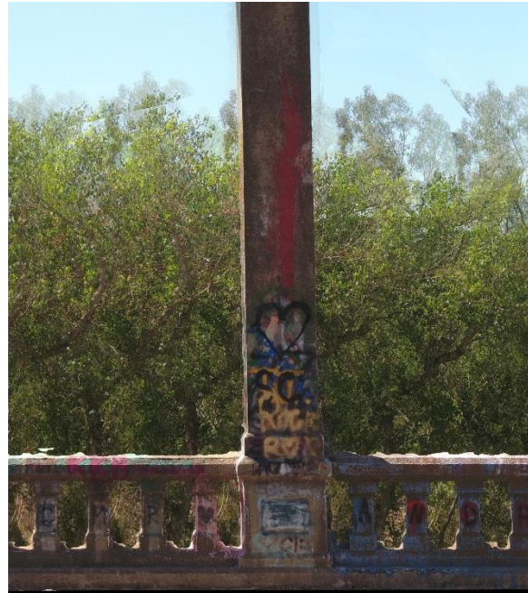
Figure 14 - Hanger 10 West borescope location
