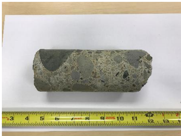
Figure 39 - Bridge Deck at Pier 4/Abutment 5 (Core 3)
