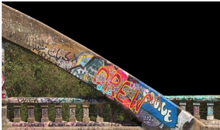
Figure 15 - Arch 3 East borescope location
