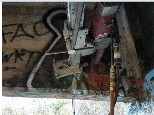
Figure 38 - West Girder (Core 4)
