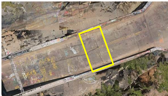
Figure 16 – GPR scan area at Abutment 1/Pier 2
