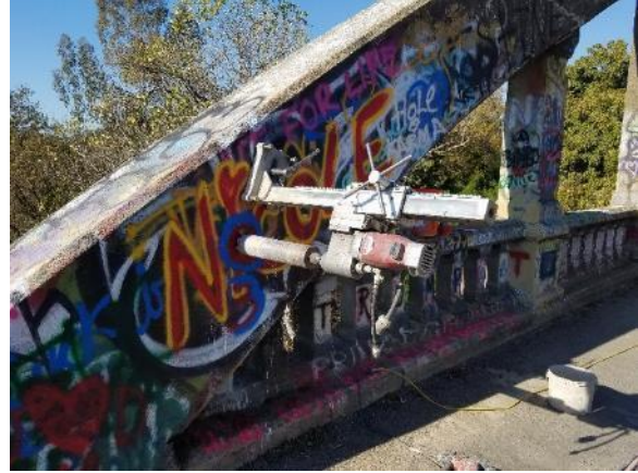
Figure 34 - Arch 3 West (Core 2)
