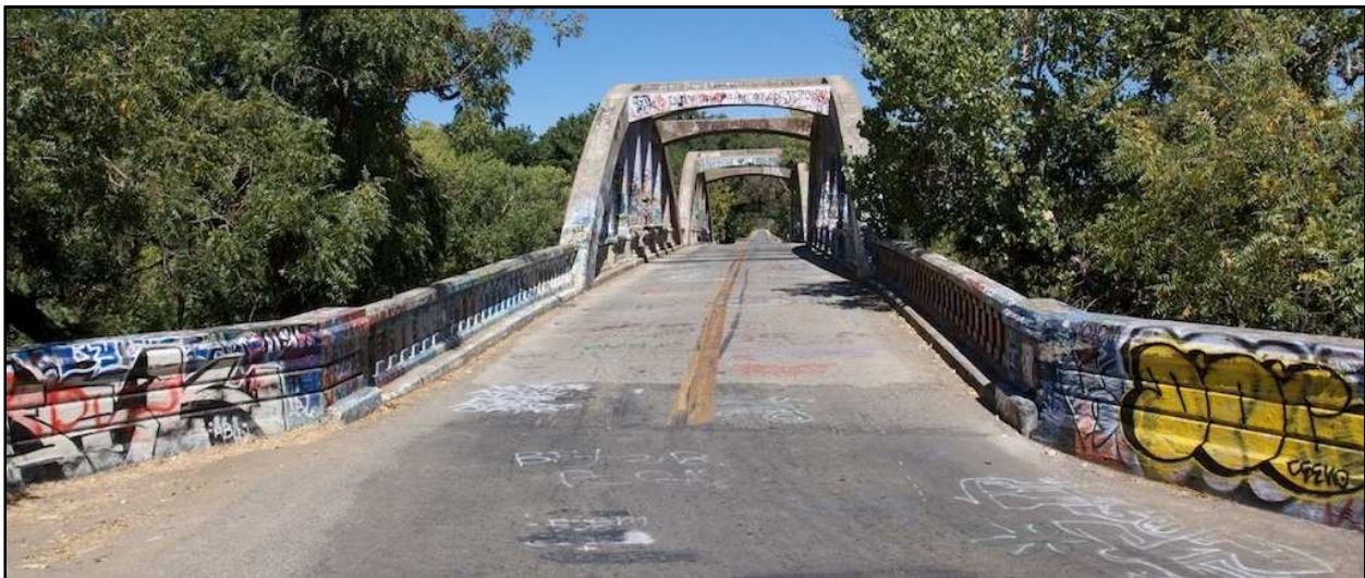
Stevenson Bridge, standing at Abutment 1, looking north
