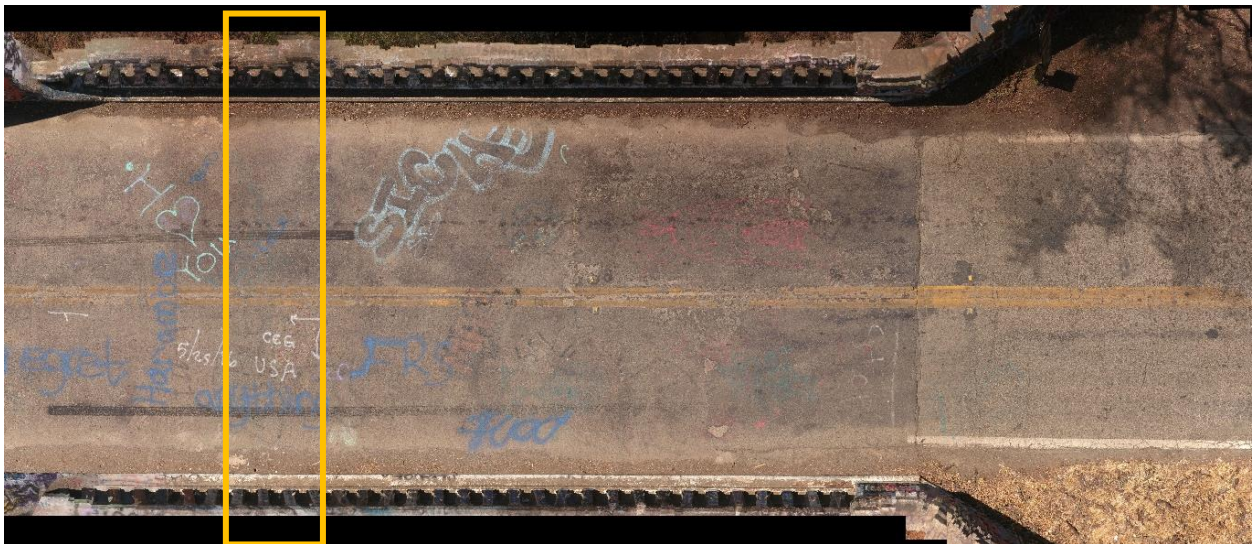
Figure 8 - Location of crack between Pier 4 and Abutment 5 as shown through UAS image
