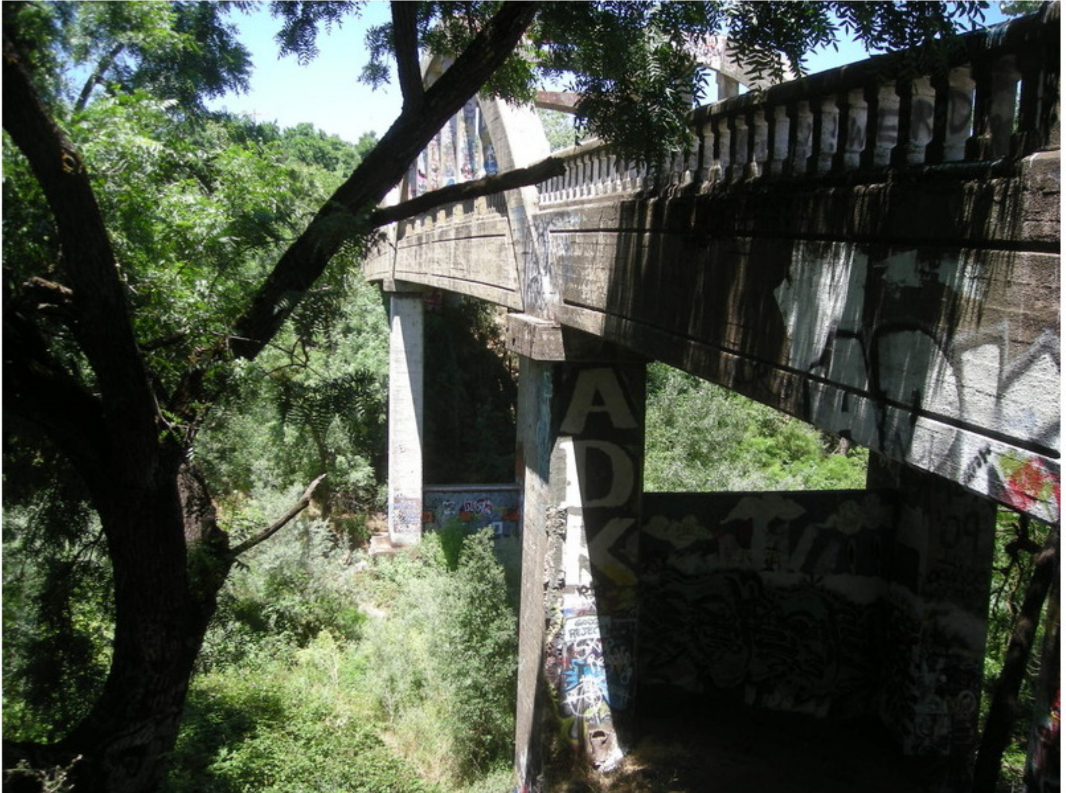
Photo No. 2 Elevation view looking Northeast
