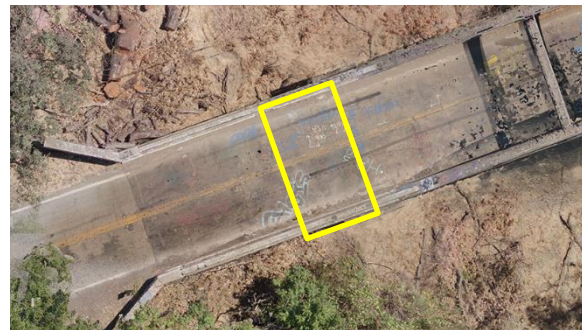
Figure 17 – GPR scan area at Pier 4/Abutment 5
