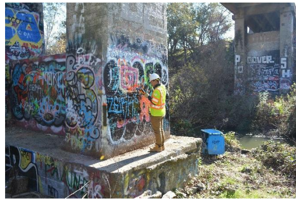
Figure 12 - Use of borescope at Pier 3 west side
