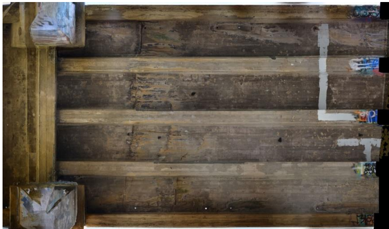
Figure 6 - Underside view at Span 1 rendered from several images
