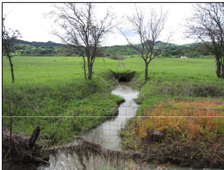
Photo 4: West Tributary to Green Valley Creek near confluence with main stem (3/7/2016)
