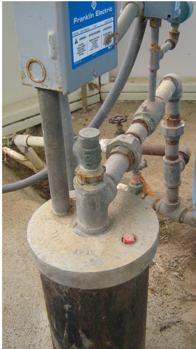
Figure 9. Photo: A domestic well showing the well casing, cover, and conveyance system.
