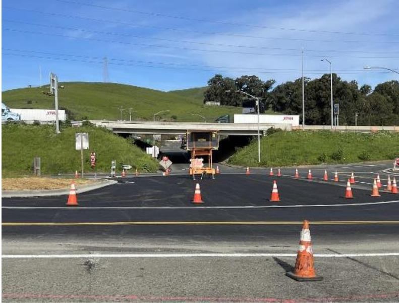
In recent weeks, construction has continued at the intersection of McGary at Red Top Road. Work included: grading the widened section and preparing the intersection for asphalt paving. The contractor is planning to switch traffic onto the newly paved Red Top Road. Please use caution when entering the construction zone and use slower speeds when equipment and crews are actively working.
