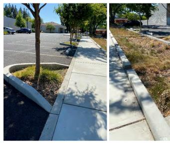
Tree Well Bioswale Bioretention in a parking lot
