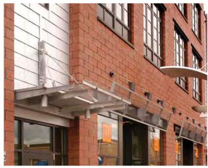
Example of appropriate building materials—brick and steel (Source: Jacobs)
