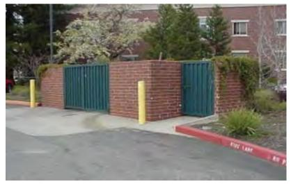
Appropriately screened service area with masonry and steel enclosure that matches the adjacent building (Source: Jacobs)
